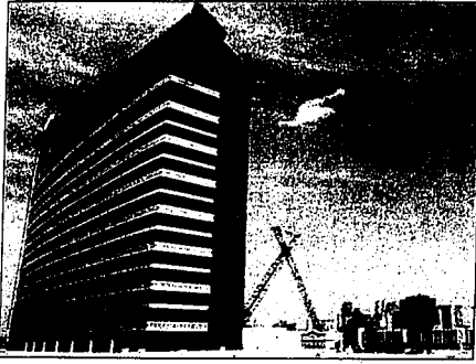
Construction is shown on the MotorCity Casino Hotel in Detroit, July 9. While getting people to think of Detroit as a regional gambling Mecca might be a longshot, casino officials and tourism promoters are working to trumpet the arrival of the city's permanent casinos to a wider audience.
