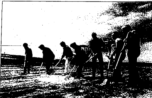
Community members and developers break ground during a Saturday ceremony for Murtaugh's first subdivision, The Legacy.
