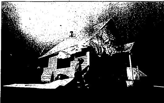
Members of the Halley Fire Department as well as the Chubbuck Fire Department wrap the Greenhorn Guard Station, which served as a ranger office from 1909 to 1920, with material to help reflect radiant heat away from the building on Saturday afternoon off Greenhorn Road south of Ketchum.
