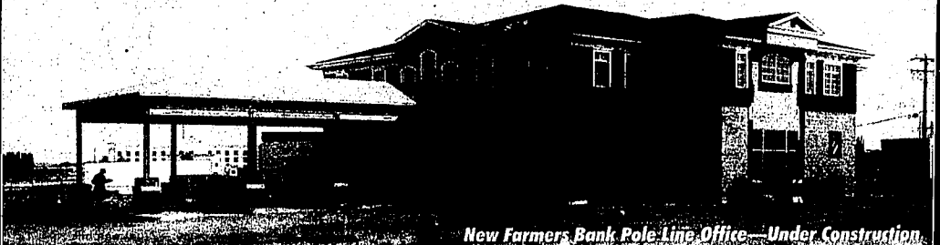
New Farmers Bank Pole Line Office—Under Construction.
