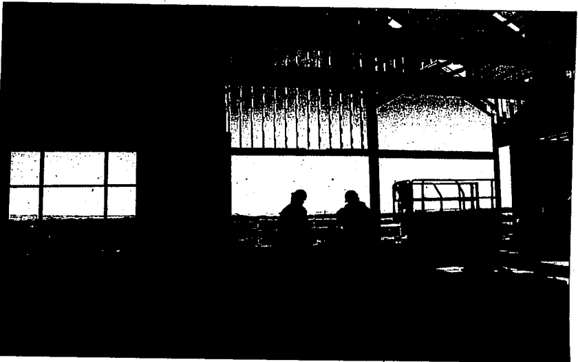
Construction workers are silhouetted against the backdrop of what will be the view from the dining room of the Canyon Crest Restaurant and Convention Center of the Canyon Rim overlooking the Snake River in Twin Falls. The building is expected to be completed in the spring of 2008.
