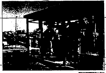
Construction workers check the inside of a smoking hut at the hospital Monday morning before it is removed from the premises as part of the transition to become a smoke-free campus.
