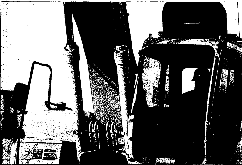
An unidentified construction worker finishes up a day of work at the Canyon Ridge High School construction site Wednesday afternoon in Twin Falls. The Twin Falls School District is proposing a facilities plant levy for up to $3.3 million annually, for 10 years. But the money would go toward maintenance on existing facilities, not the construction of the new high school.
