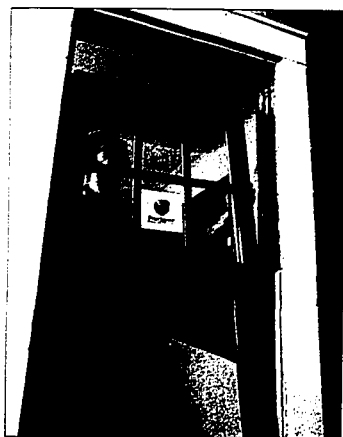
This aluminum-clad wood replacement window can have efficient low-emissivity glass with a special coating for easy cleaning.
