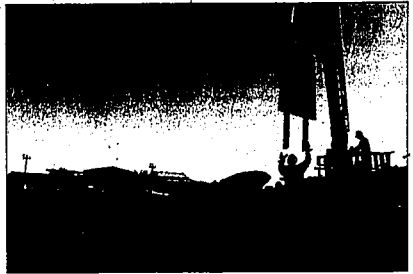
Bruce Spratt of Lytle Signs guides one of the new metal signs for The River Christian Fellowship as Travis Tucker mans the crane Friday afternoon at the Twin Falls church. According to the Rev. Mike Kester, the change of name was about the only difference the congregation noticed as River Christian severed ties last year with Calvary Chapel, a national nondenominational Christian church.
