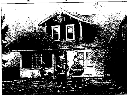
An electrical fire broke out Tuesday morning in the childhood home of former Declo resident J.R. Simplot. It burned more than half of the upper story and caused extensive water damage to the rest of the house. The family currently residing in the home was not injured.
