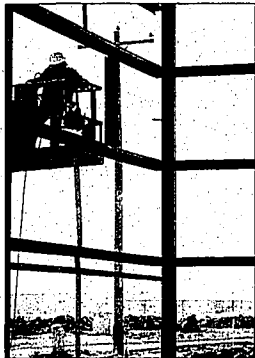
Mike Whiteman, an employee with Starr Corporation, installs structural steel at the Robert Weid Plywood Corporation construction site Monday afternoon in Twin Falls.
