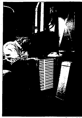
With its great thickness as compared with standard fiberglass filter, a pleated media air cleaner usually requires professional installation for the duct modifications needed.
