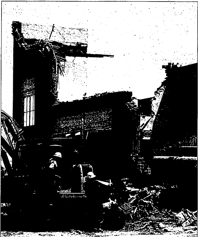
Employees of Ideal Demolition Service proceed with the demolition of the old Kimberly School Wednesday afternoon in Kimberly. The school, which was approved by a bond issue passed in 1914, according to Kimberly School Board Chairman Dave Fullmer, has been out of use since 2001, when the new Kimberly High School opened. "It's a strange feeling for me, a chairman of the board, to have been in high school in that building and be responsible for that removal," Fullmer said. "But it's become a liability to the district and an unusable space. Overall, I think it was past due."
