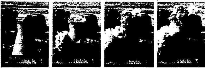
The demolition of the 60-foot-tall cooling tower is shown at the main reactor complex in Yongbyon, North Korea, on Friday. North Korea destroyed the most visible symbol of its nuclear weapons program Friday in a sign of its commitment to stop making plutonium for atomic bombs.
