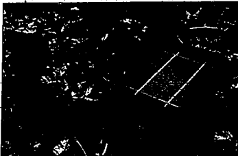
This remote solar panel powers three spotlights on long wires. Three rechargeable batteries are located in the solar cell panel housing.
