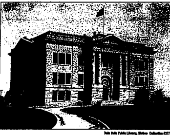
The Twin Falls County Courthouse, completed in 1911, once housed the Twin Falls Public Library (you can see this on the ground window on the left-hand side of the building). In the spring of 1912, the courthouse allowed the library to move in. Since the county was helping to pay for some of the library's operating costs, county residents were able to get free cards. However, a year and a half later, the county needed the space the library occupied, and county residents lost the privilege of using the library for free. By 1913, the library owned 2,000 books (up from 150 books in 1909), and about 1,000 books circulated each month. Both the library and the courthouse are coming up on their 100-year anniversaries.
