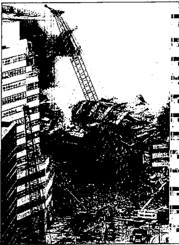
A crane looms over the smoldering wreckage of World Trade Center building 7 in New York on Sept. 18, 2001. Federal investigators said Thursday they have solved one of the mysteries of the Sept. 11 attacks: the collapse of World Trade Center building 7, a source of long-running conspiracy theories.
