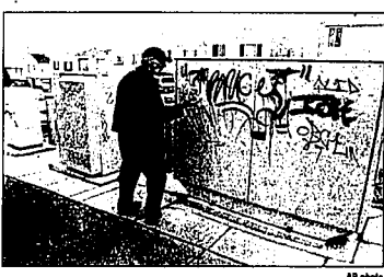
David Crommie, president of the Cole Valley Improvement Association, looks at an AT&T serving area interface (SAI) box in San Francisco, Tuesday. The cabinet in the middle is a U-verse VRAD cabinet and the far left cabinet is a power transfer switch (PTS). Crommie said AT&T received an exemption from environmental review to install up to 850 cabinets in San Francisco, which his group opposed.
