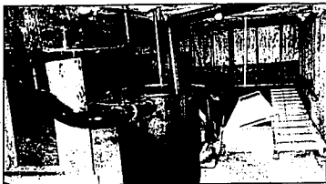
Main greywater collector unit tank with plumbing leading to it from the various greywater sources in the house.
