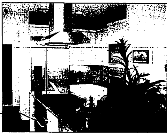
This island-style range hood can communicate with a fresh air ventilation system to provide outdoor fresh air to the house when the range hood is running.
