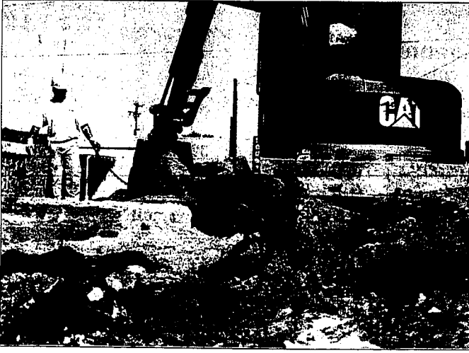
A section of the torn-up South Lincoln Street sidewalk in Jerome awaits reconstruction as Gordon Paving workers Robert Hanson, left, and John Kober, operating a CAT backhoe, work to remove old piping from the site. Work is underway to reconstruct falling areas of sidewalk on both South Lincoln Street and Main Street.
