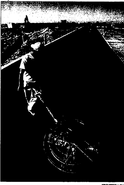
Brock Trudy, with Petersen Brothers Construction Inc, works on the expansion of Rite Stuff Foods Tuesday in Jerome. The food processing company is expanding its production capabilities as well as diversifying its product line.
