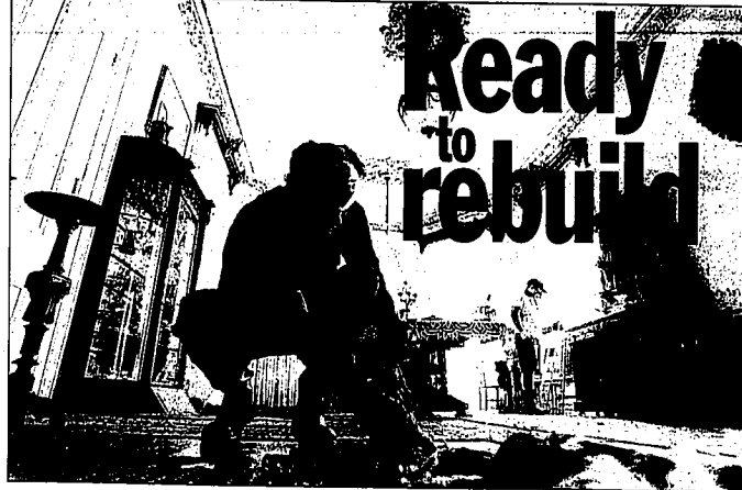
Lyman Labry rips out flood-damaged carpet out of Ashton Villa, a building that survived the killer storm of 1900, in the aftermath of Hurricane Ike, in Galveston, Texas, Thursday.
