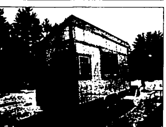
Elizabeth Turnbull's 'Tiny House' is being constructed on the grounds of her alma mater, The Governor's Academy prep school in Byfield, Mass. Turnbull is building her 6-foot-by-18-foot rolling home using state-of-the-art green materials; it will be powered by solar panels. Turnbull hopes to live in the home during her two years studying at the Yale School of Forestry and Environmental Studies.
