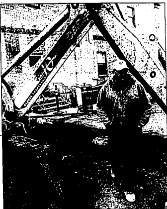
Scott Roth, owner of Loma Land LC of Rupert, looks over an excavation site for a new water line in between the Minidoka County Courthouse and the Minidoka County Sheriff's office Monday.
