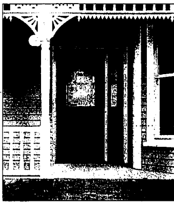
Frosted glass in an insulated steel door provides natural light without sacrificing privacy and security.
