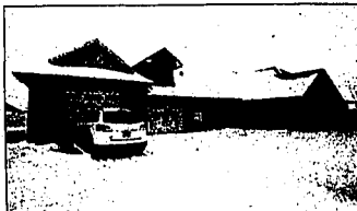
Robert Ramos's Twin Falls home took eight months to complete.
