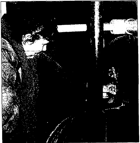
La Dea Miller checks pressure in one of the big filters in the downstairs machine room at the pool on Thursday.
