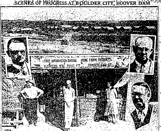
Here are scenes at Boulder City, Nev., construction site for Hoover Dam. Above, what will be the industrial region of the 250,000 m. city; below, first to capitalize the lucrative life of tourists and workers were Mr. and Mrs. W. P. Elliott, proprietor of Boulder City, and Mr. and Mrs. J. C. Walker, chief engineer, both of the United States reclamation service; below, Louis C. Grandon, government appointed 'father' of the city.
