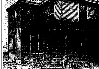
Old houses like these are a drain on the pocket book of the owner. They stand neglected and in a sorry state. After this house was modernized it was again photographed as shown above.
