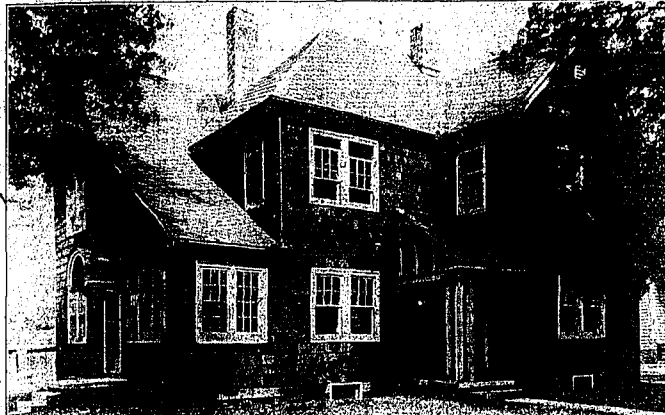
No one wanted to rent this house as it originally appeared. But when it was modernized... it's rented now.
