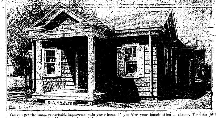
You can get the same remarkable improvements in your house if you give your imagination a chance. The trim little cottage above was once the old, worn-out home below.
