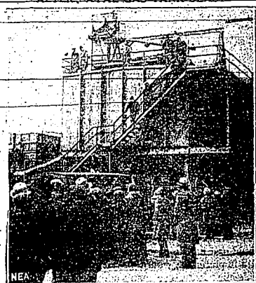
AFTER FATAL GAS-TANK BLAST
