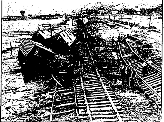
Prayers of Iowa farmers for rain were answered a hundredfold when the heavens gushed and damaging floods swept the state, parched by months of drought. Here is a remarkable picture of the toll taken by deluge, the wreck of a train, cut off by washout of tracks near Council Bluffs, Ia., when Henry creek became a raging torrent overnight. With cars spilled from the rails and flood debris littering the tracks, workmen are toiling to reopen the way for trains.
