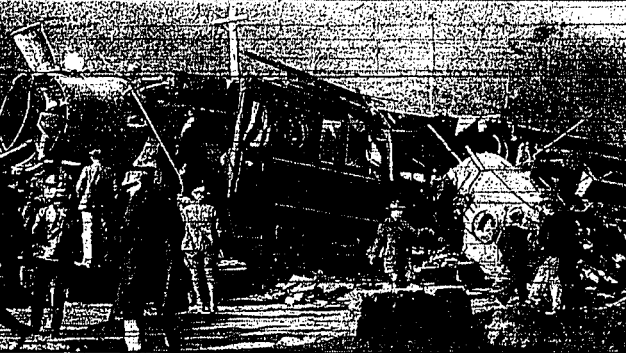
The shattered engine, its interior tipped out, leaving only a steel shell; the ruin of the locomotive boiler, lying at the right; and a car torn almost in two by the blast are the ghastly reminders of the lives of 16 miners and two engineers who perished in a mine train blast on Tuesday night. The train was carrying 350 persons to the pits of the Killbuck-Murray coal mine, when the boiler exploded and the train was sent hurtling toward the engine, which was the last survivor.
