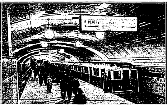
A monumental feat in construction speed and engineering skill achieved by the Soviet government, the great Moscow subway, nearly eight miles long, is traversed daily by thousands of passengers on its recent opening. This picture gives striking evidence of the effort to make it the most beautiful underground traffic artery in the world. The Lenin Library station, shown here, has striking lighting effects, lofty vaulted ceilings, and walls and pillars decorated with marble in varied colors.
