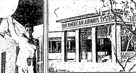
Modern hotels, equipped to accommodate passengers and crews and their stores, have been built at Clipper bases across the Pacific. Above is the Pan American Airways Inn, a new part of the Wake Island skyline. At left, a Pan American Airways airplane is being refueled at Wake Island. This information is relayed to Clipper pilots at the relay station.
