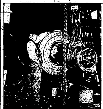
One of the two drive shafts for the America. Just enough is exposed for attaching the huge propeller.
