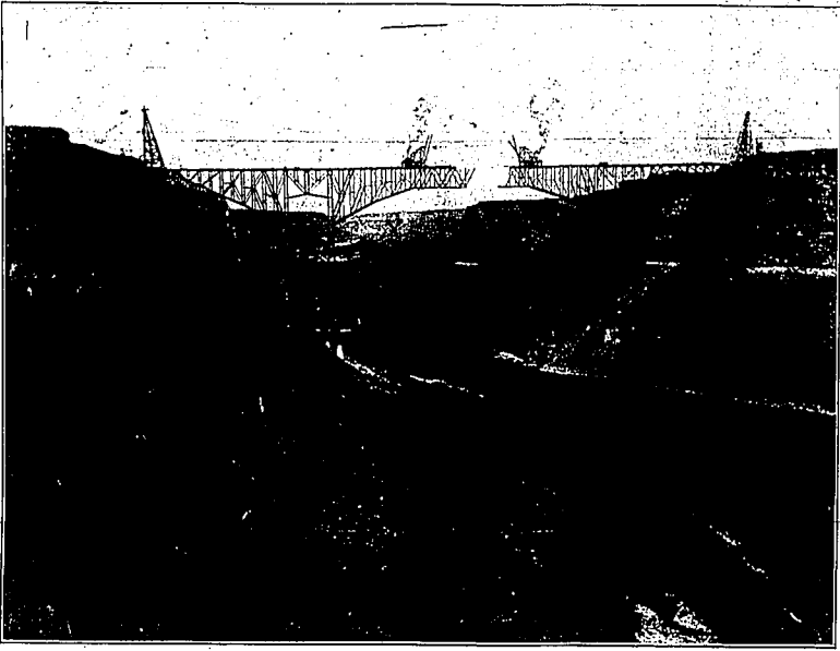
This view of the Twin Falls-Jerome Intercounty bridge which was photographed just 18 days before the floor was laid so that the first car could be driven across the span in September, 1927, shows steel bolts shown far out over the structure were used to lift great steel girders and beams into place as fabrication of the mighty span proceeded apace.
